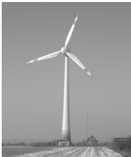
Figure 1. 4.5 MW horizontal-axis wind turbine type E112, selected for operational load monitoring using fibre-optic sensor technology. Photograph: Enercon GmbH.
