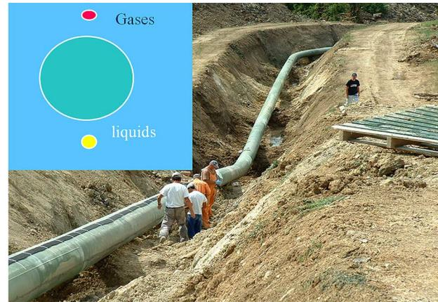
Fig. 20. Fluid leakage detection in pipelines using fiber distributed sensing technologies. Inset: illustration of situation of fiber cable transducer (in relation to the pipeline) for gases and liquids. Photo: installation of the transducer cable on a pipeline. Courtesy of D. Inaudi.
