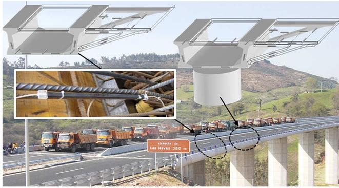
Fig. 18. 35 lorries with 35 tons each during the load test of Las Navas viaduct on the A8 motorway, in Cantabria, Spain. The insets show one of the transducers during its installation, and two sections where the transducers were embedded. Courtesy of the PhotonicsEngineering Group at the University of Cantabria.
